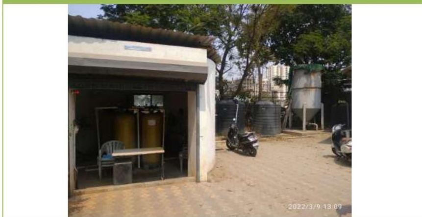
Sewage Treatment Plant (STP)
